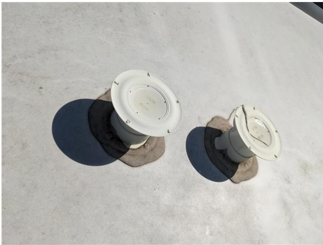
17.7 Item 1 (Picture) Plumbing vents
