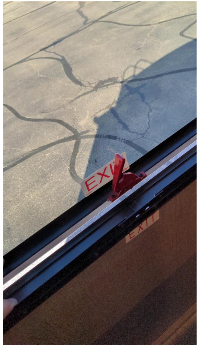
22.13 Item 2 (Picture) emergency exit window confirm operation
