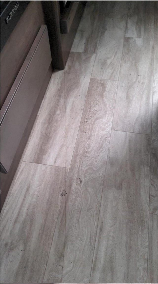
1.1 Item 7 (Picture) floor staining near stove
