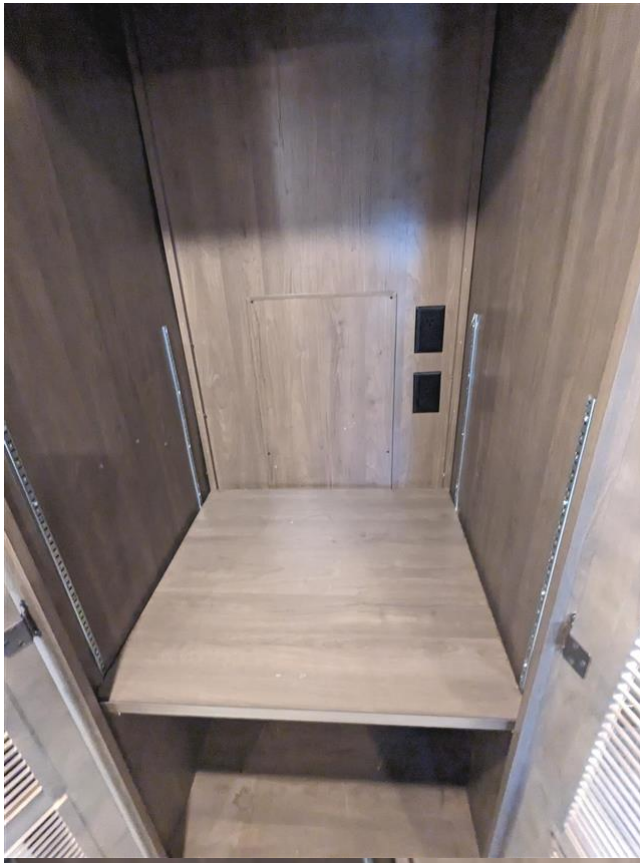
18.11 Item 1 (Picture) Closet plumbed for W/D
