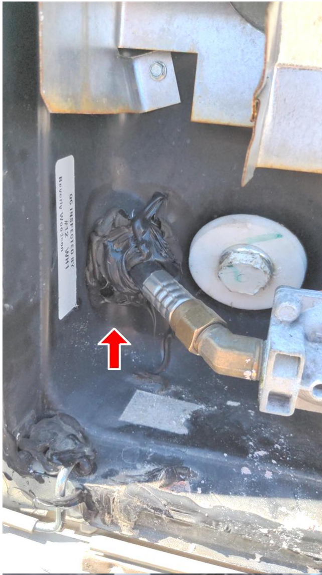
13.1 Item 1 (Picture) water heater grommet sealed
