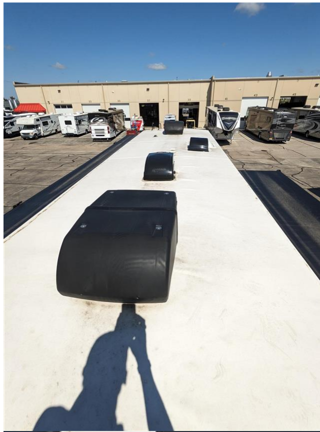
17.0 Item 2 (Picture) Roof - Front to Back
