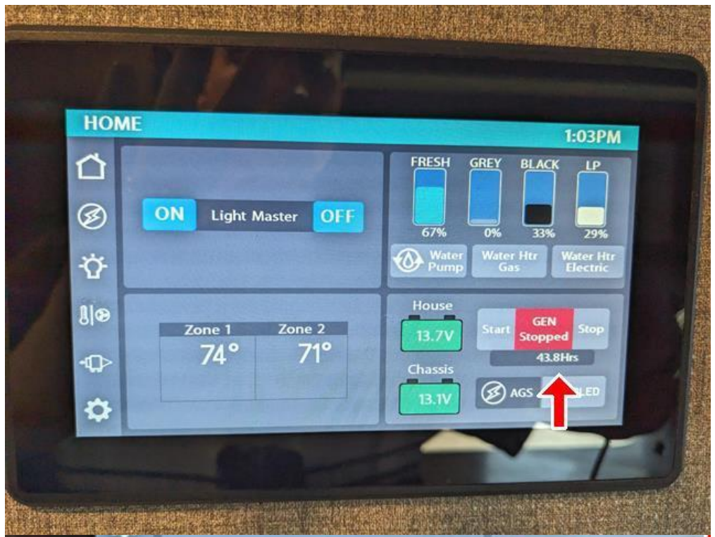
16.18 Item 5 (Picture) Generator Hours = 43.8
