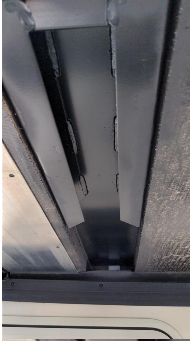
12.3 Item 4 (Picture) Slidell floor detail too
