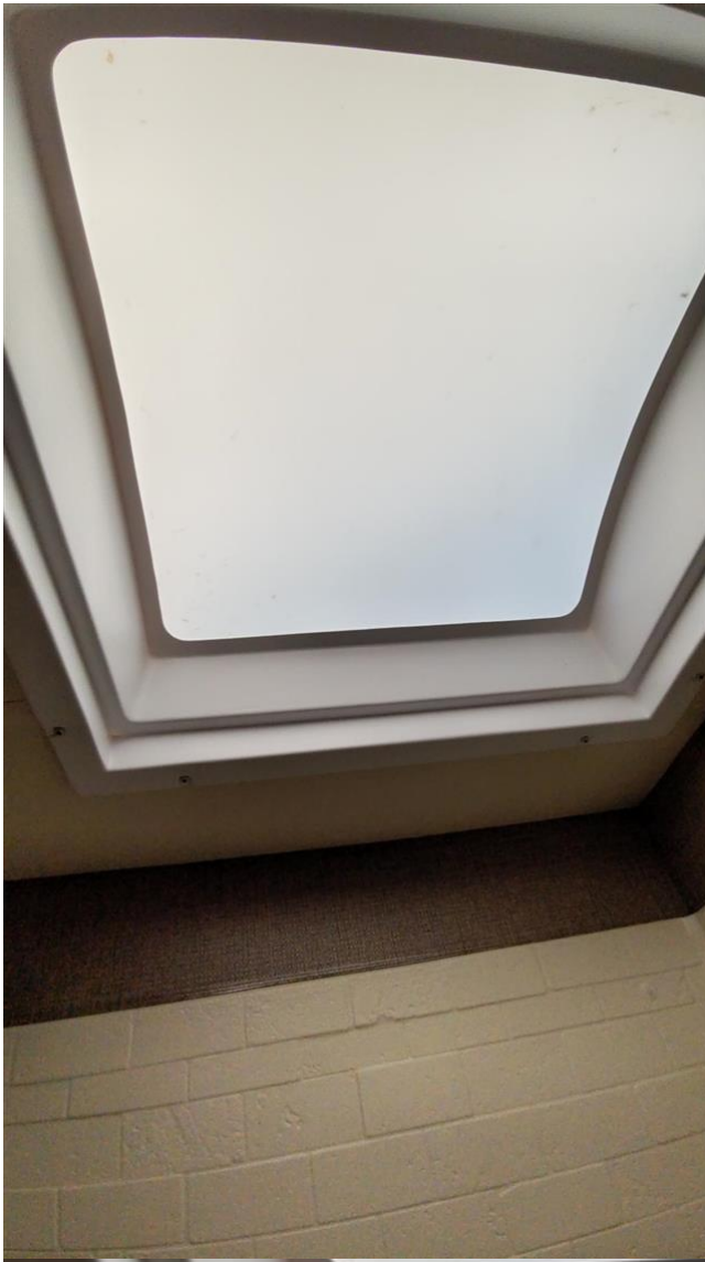
20.5 Item 1 (Picture) skylight
