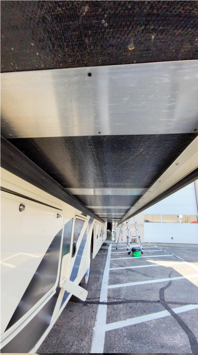
9.4 Item 4 (Picture) slide out floor
