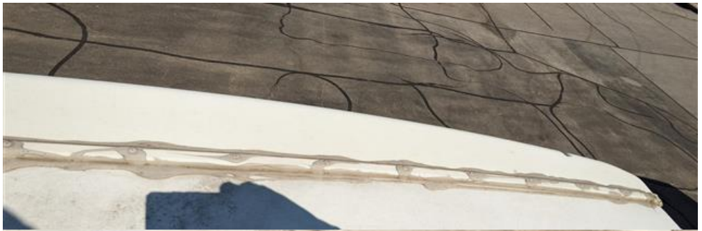
17.1 Item 3 (Picture) Lap Sealant
