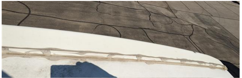
17.1 Item 3 (Picture) Lap Sealant
