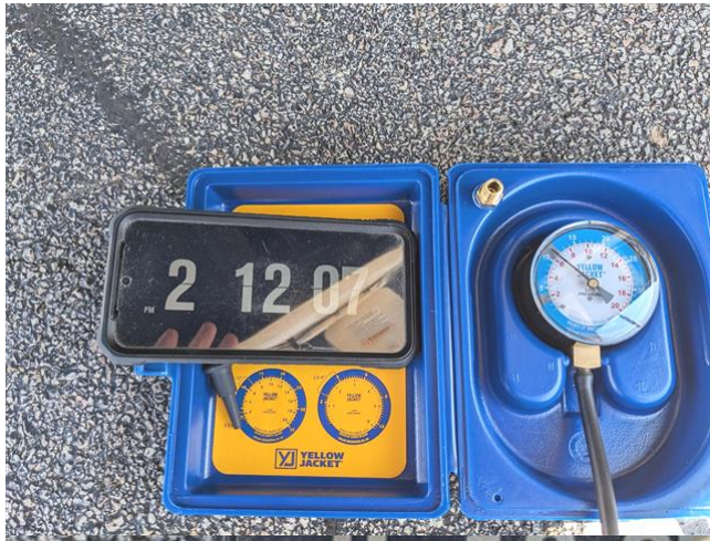
19.0 Item 1 (Picture) Begin
