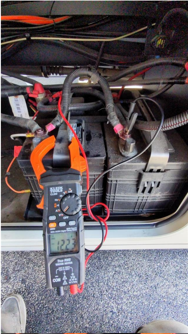
16.11 Item 2 (Picture) Coach battery voltage while on generator
