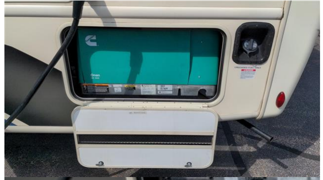
11.5 Item 2 (Picture) rear generator compartment
