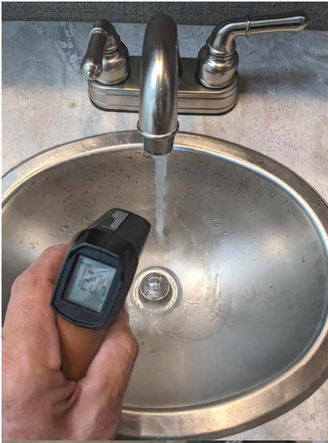
18.2 Item 1 (Picture) Hot water temperature
