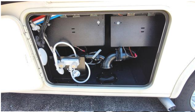
14.0 Item 1 (Picture) water bay overview
