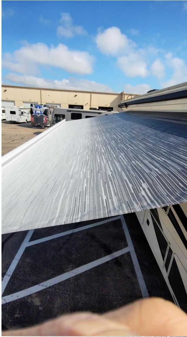
7.0.A Item 2 (Picture) awning fabric on top
