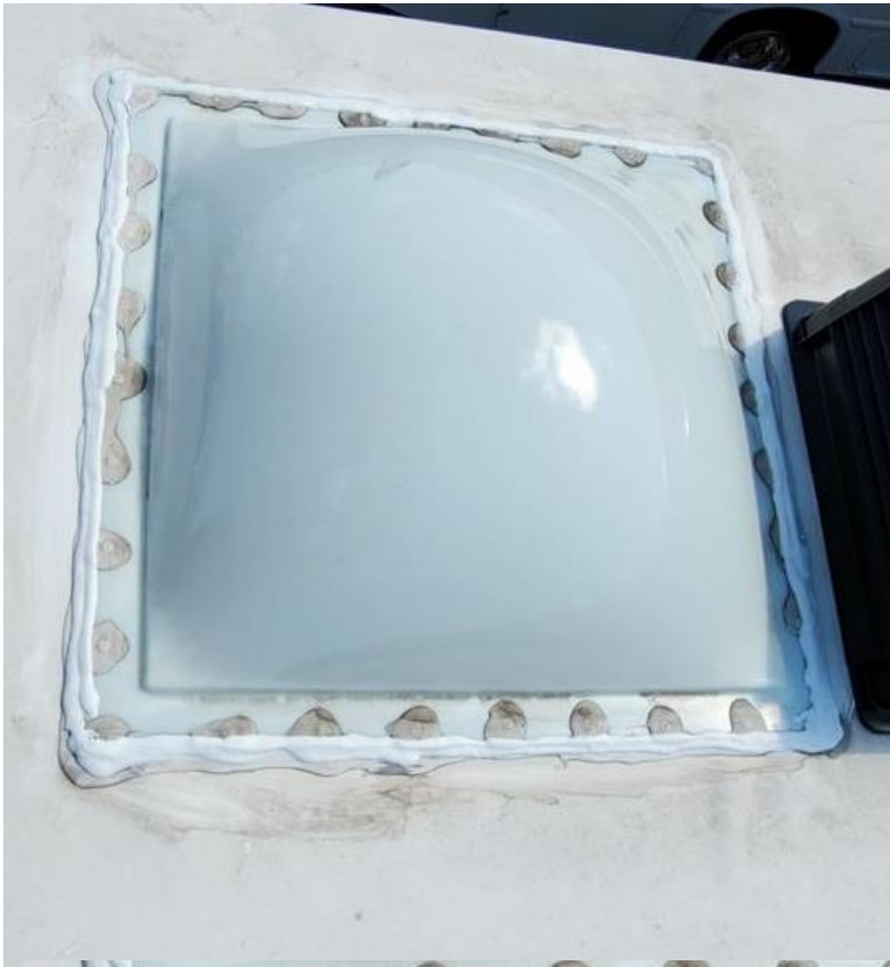
17.9 Item 1 (Picture) Resealed lap sealant
