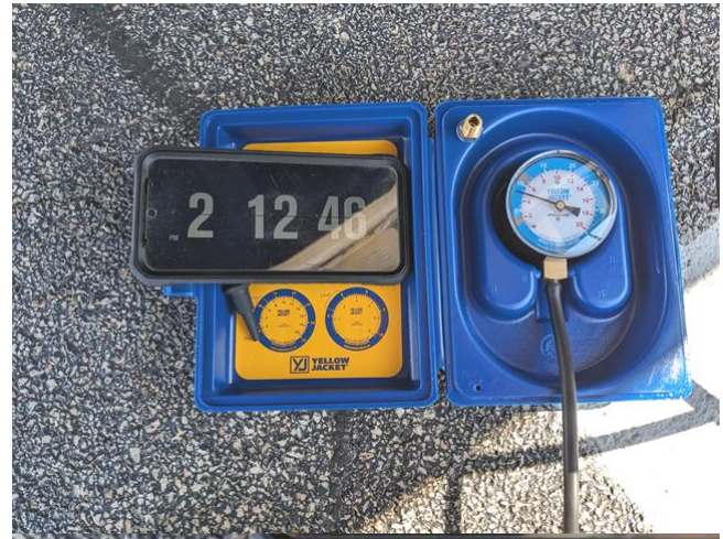
19.0 Item 2 (Picture) Bled down to 8
