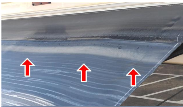
7.0.A Item 3 (Picture) faded awning fabric at upper edge
