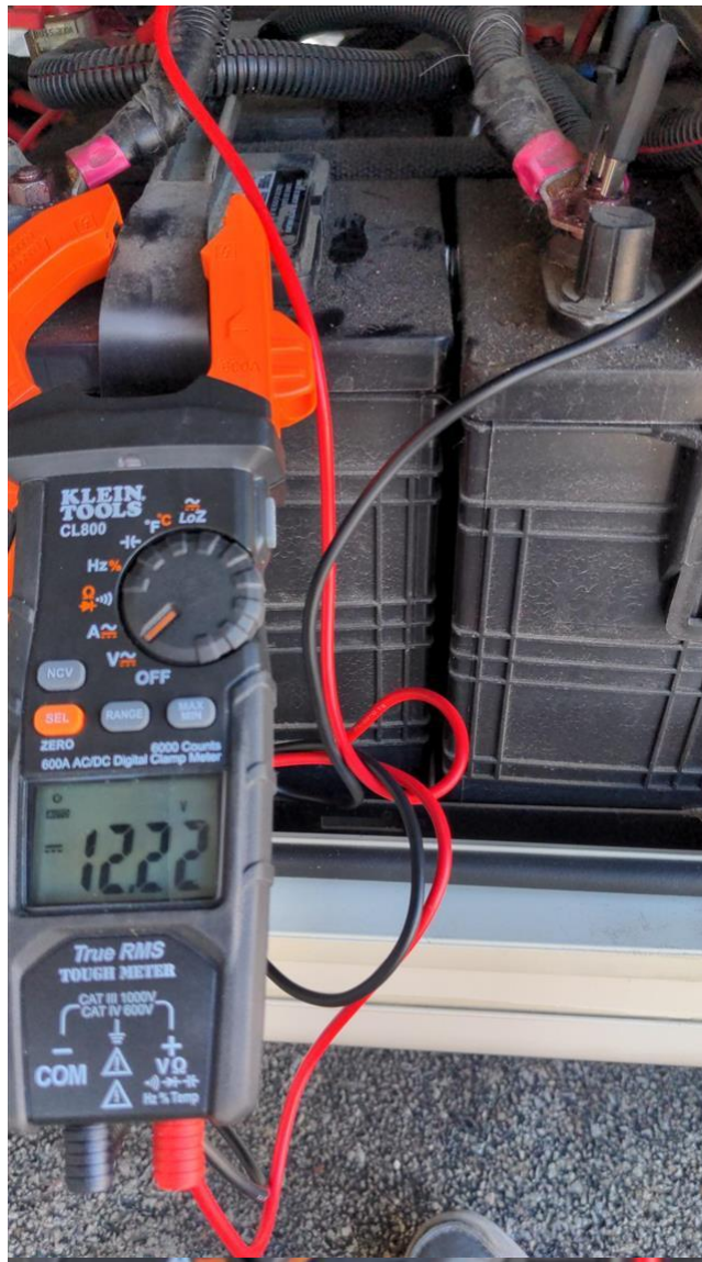
16.6 Item 2 (Picture) battery voltage external power off
